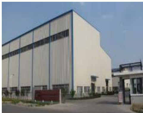
Cemtek Tianjin Machinery
